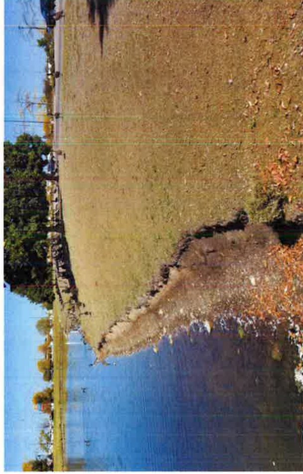
Turf Grass Pond - Severe shoreline erosion
